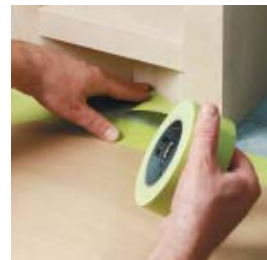
Masking surfaces for lacquer coating application
