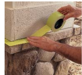
Masking concrete
