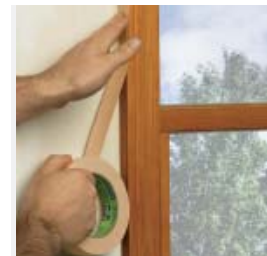
Masking window trim
